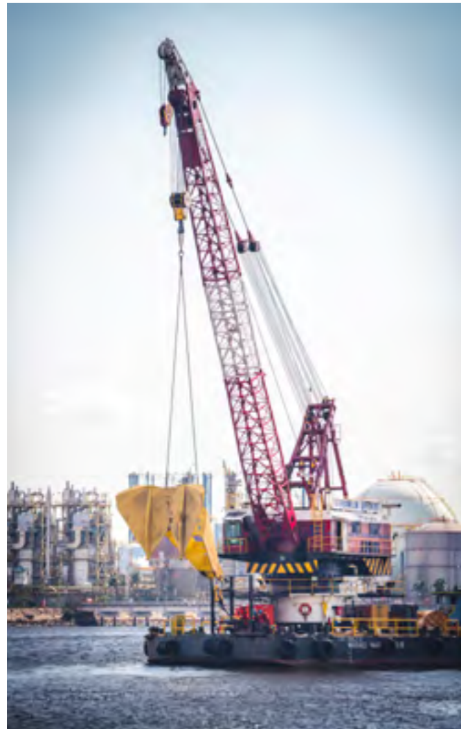
Wakaei Maru No. 8 100 Tonne Crane Barge
